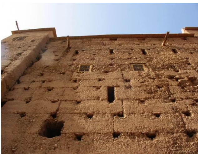
Figures 3 and 4: Examples of rammed earth (left) and earthen brick (right) walls in the ksar of Tamnougault
