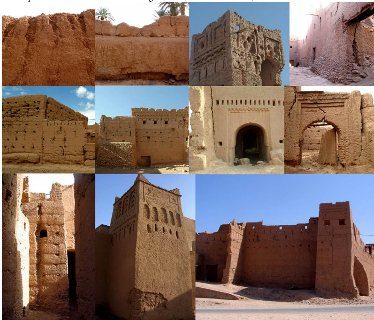
Figure 11: Principal pathologies of the earthen buildings of the Drâa valley.
