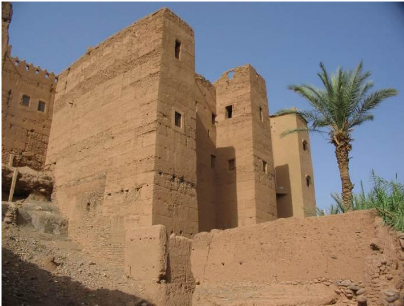
Figure 6: Rammed earth masonries of a Kasbah in Tamnougault (left).
