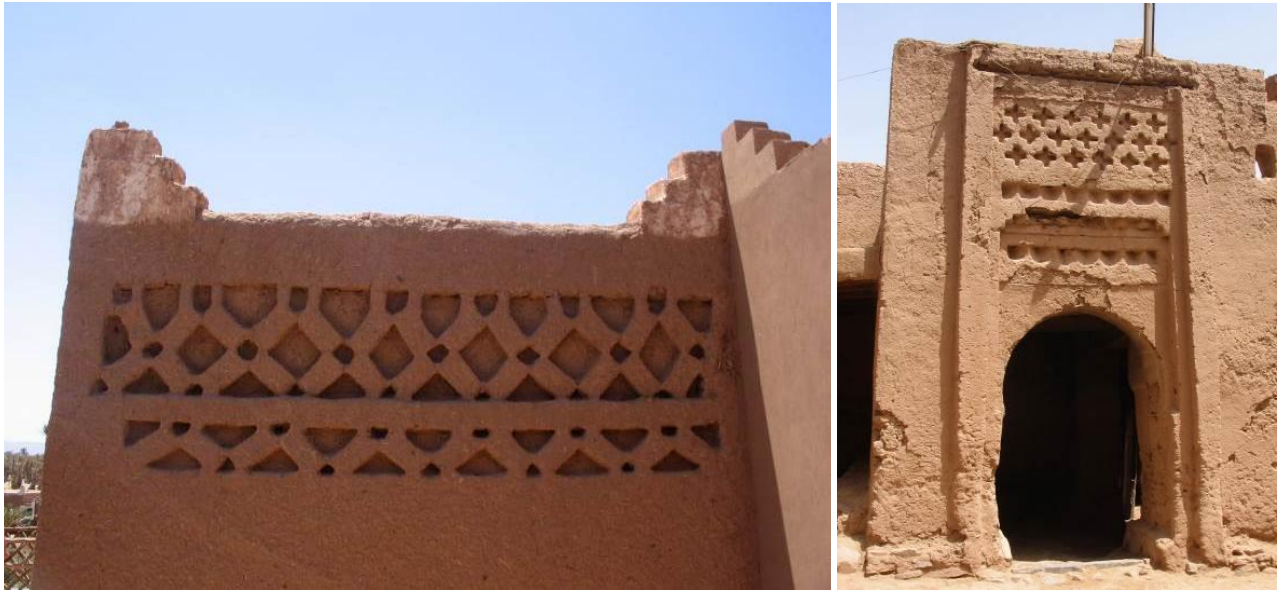
Figures 8 et 9: Examples of a decoration made with earthen brick masonries in Tamgrout and Tissergat ksour.
