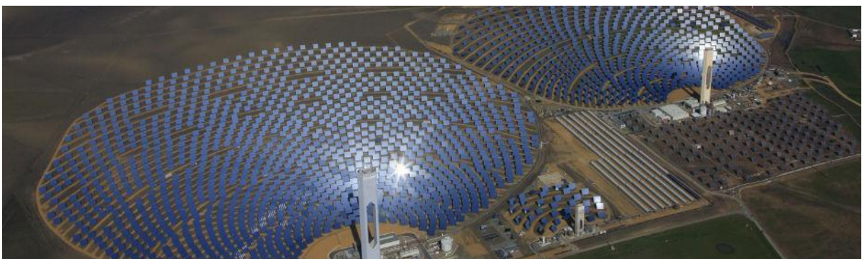
Figure 5. An 11MW and 20MW Solar Thermal Plant, Solar Platform, Sanlúcar, La Mayor, Seville Province, Spain Source:( Taylan and Berberoglu 2013 )
