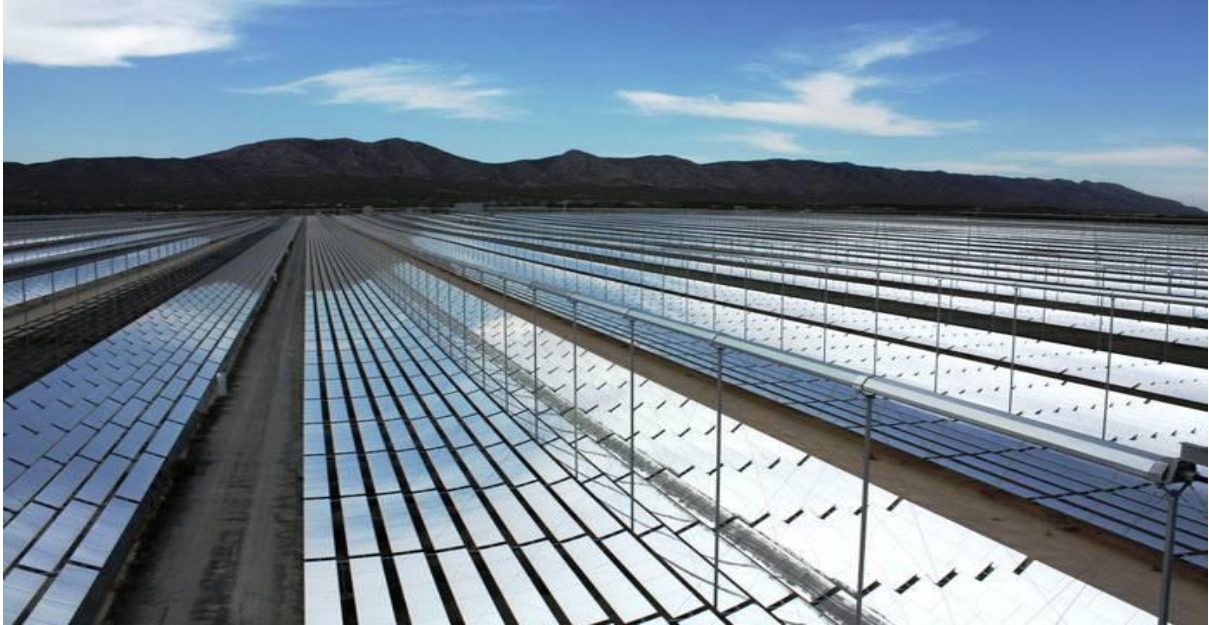
Figure 4. A 30MW Linear Fresnel Reflector System Puerto Errado 2 Thermo-Solar power plant (PE 2) at Calaspara Spain Source:( Taylan and Berberoglu 2013 )
