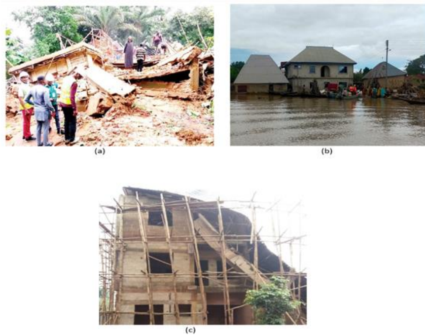
Figure 2. Sample images of building collapse caused by different variables, (a) poor foundation, concrete mixture, and quality of materials (Obianeri, 2023), (b) flood/heavy downpour (Elekwa and Oota, 2022), and (c) delay in completion of buildings under construction/aged building (Editor, 2021).
