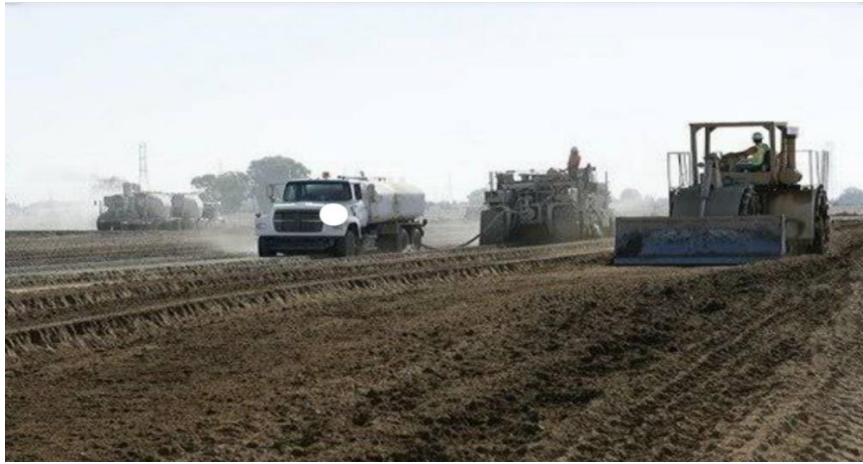
Fig. 4.3 Subgrade Stabilization with Lime.
