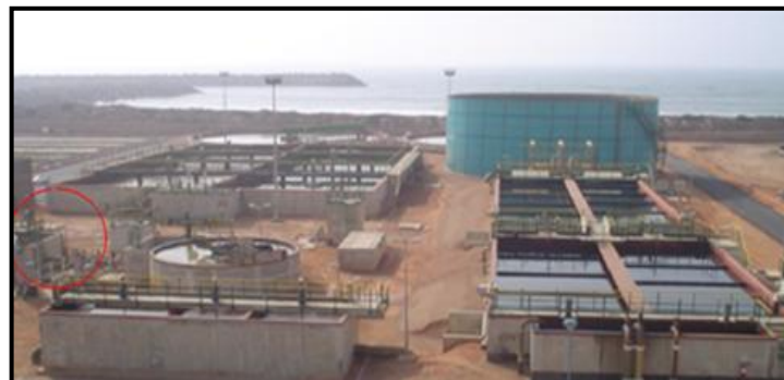
Figure 2: SAMIR wastewater treatment station
