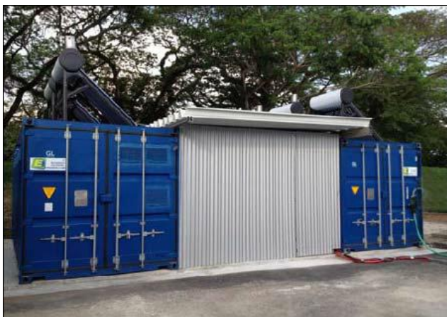
Figure 1. The modular concept of the MBPP, is in prefabricated design and can be installed easily.
