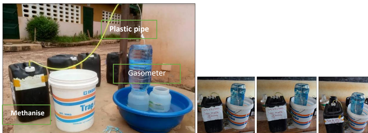
Figure 3 : Actual installation of the biodigester and gasometer
