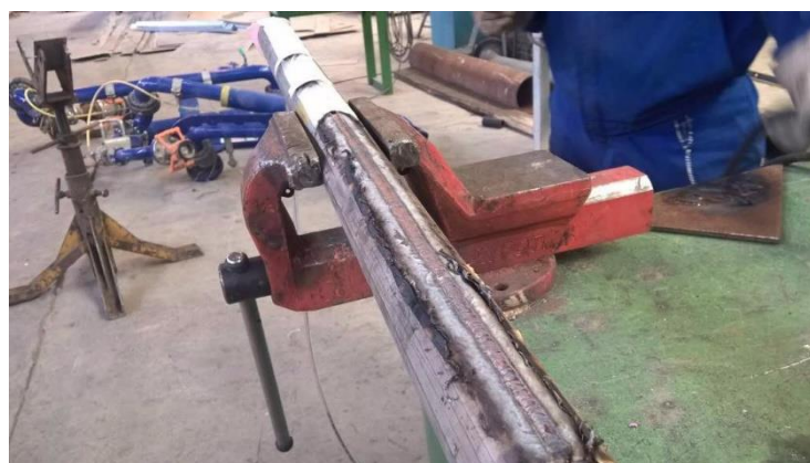
Figure 3. Welded pipe before cleaning.
