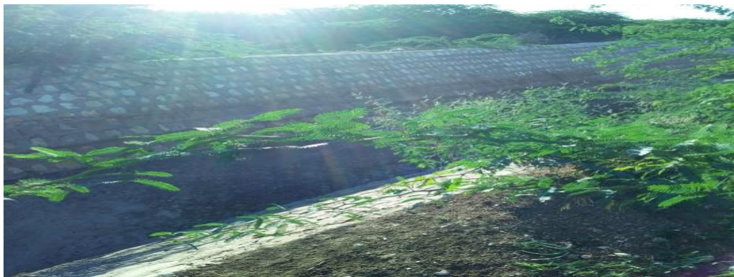
Figure 5: Infested irrigation canal at Mara,ato canal
