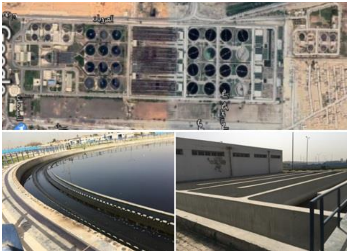
Figure 1: Berka wastewater treatment plant (Egypt)
